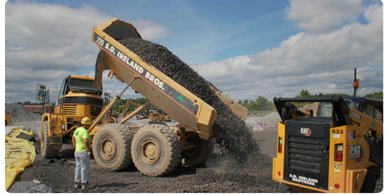
Geotextile and foamed glass aggregate placement
