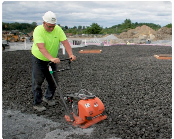
Plate compactor compaction
