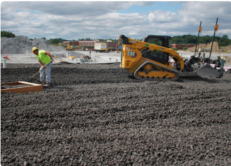
Tracked equipment compaction
