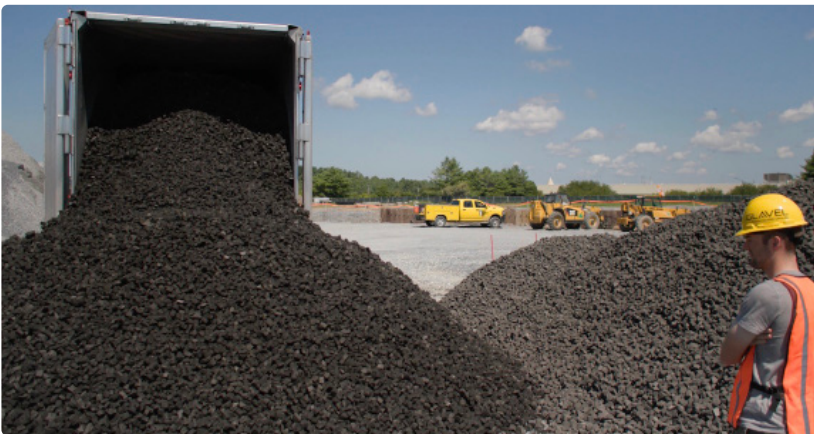
Placement and compaction of foamed glass aggregate
