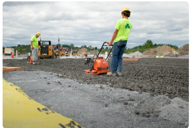
Placement and compaction of foamed glass aggregate
