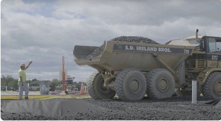
Geotextile and foamed glass aggregate placement
