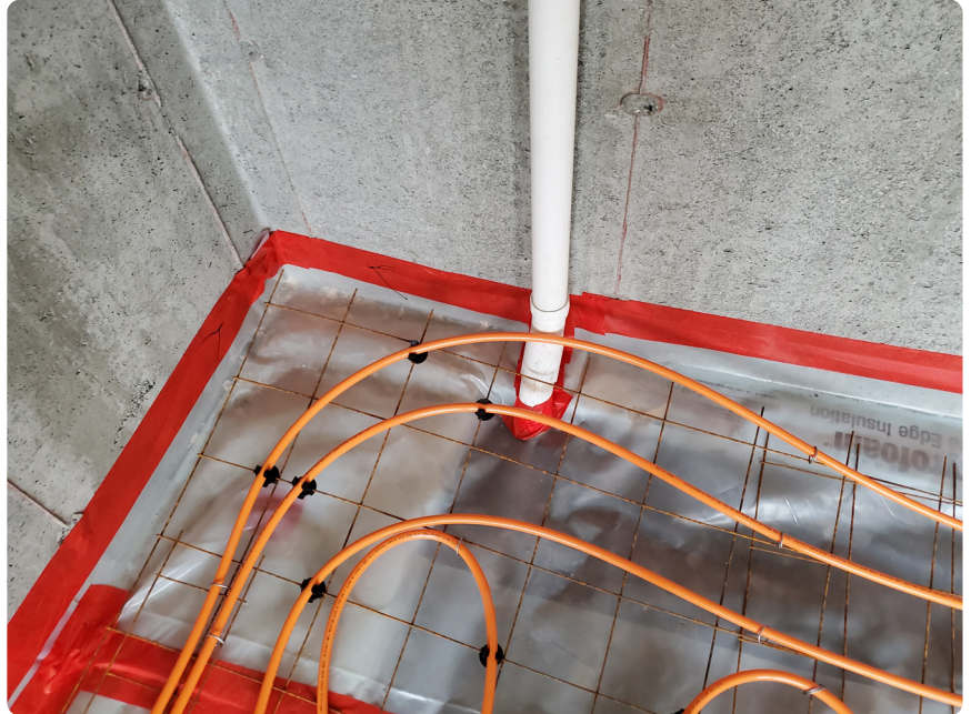
Vapor barrier with radiant heat
