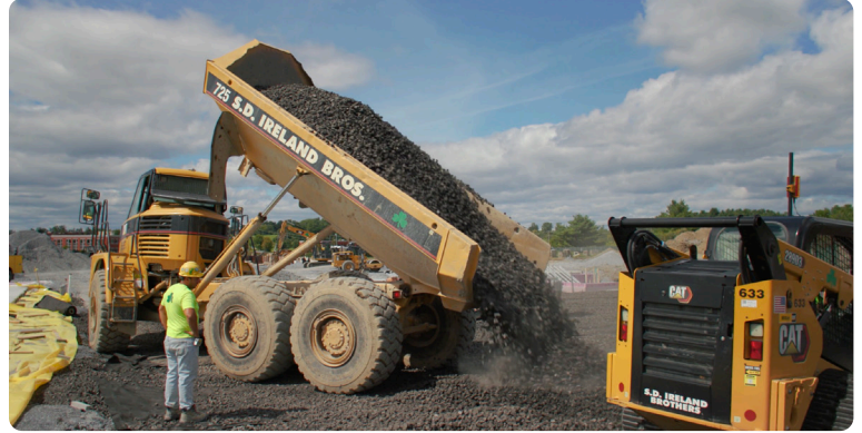
Geotextile and foamed glass aggregate placement
