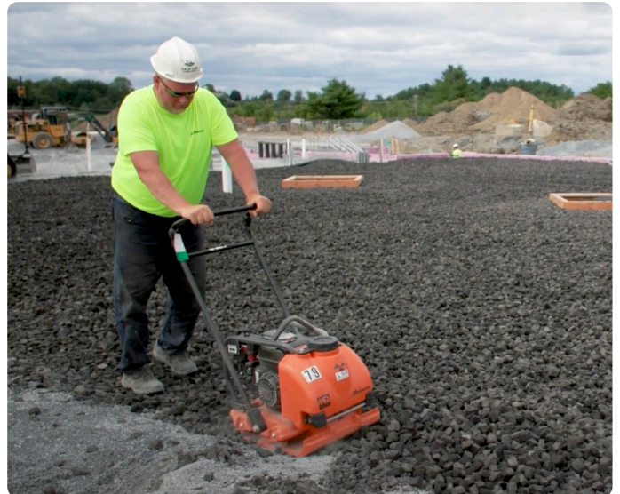
Plate compactor compaction
