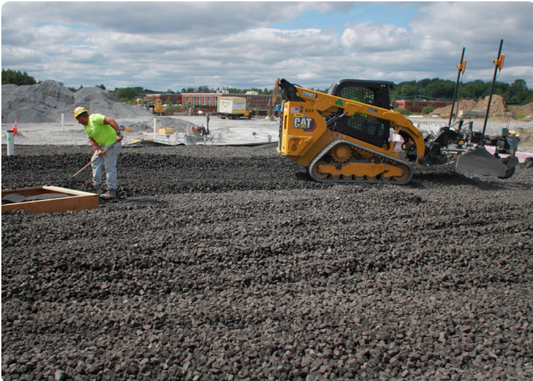
Tracked equipment compaction
